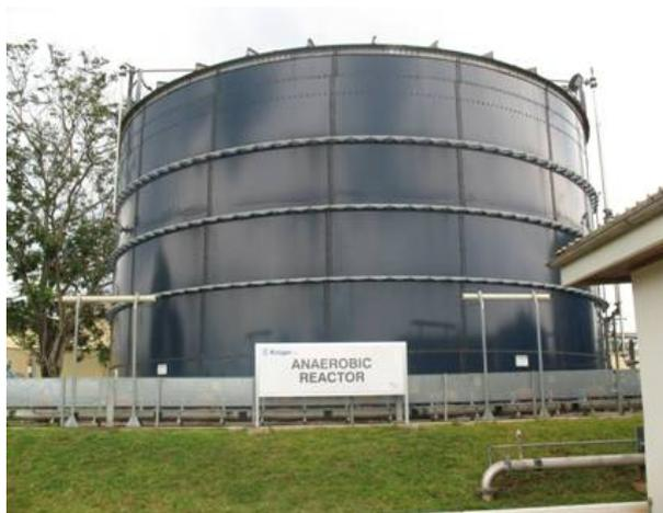
Figure 11. An 800 m<sup>3</sup> UASB bioreactor at Guinness Ghana Breweries Limited, Kumasi, August, 2008
