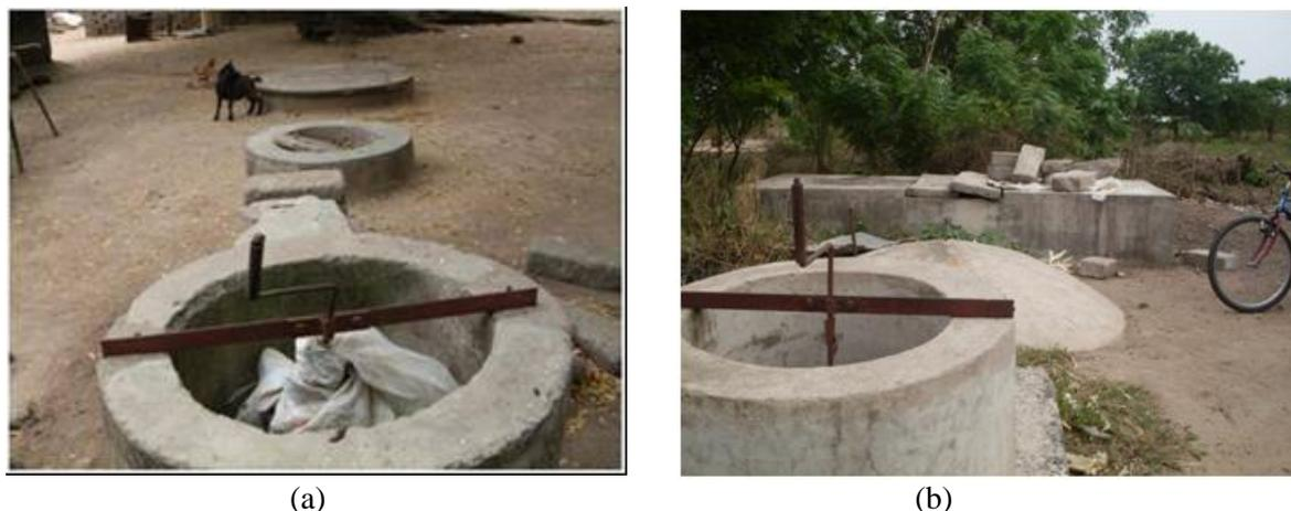
Figure 7. (a) Remains of a Chinese dome at Applonia, February, 2009, and (b) A broken-down Deenbandhu digester at Okushibli; February, 2009
