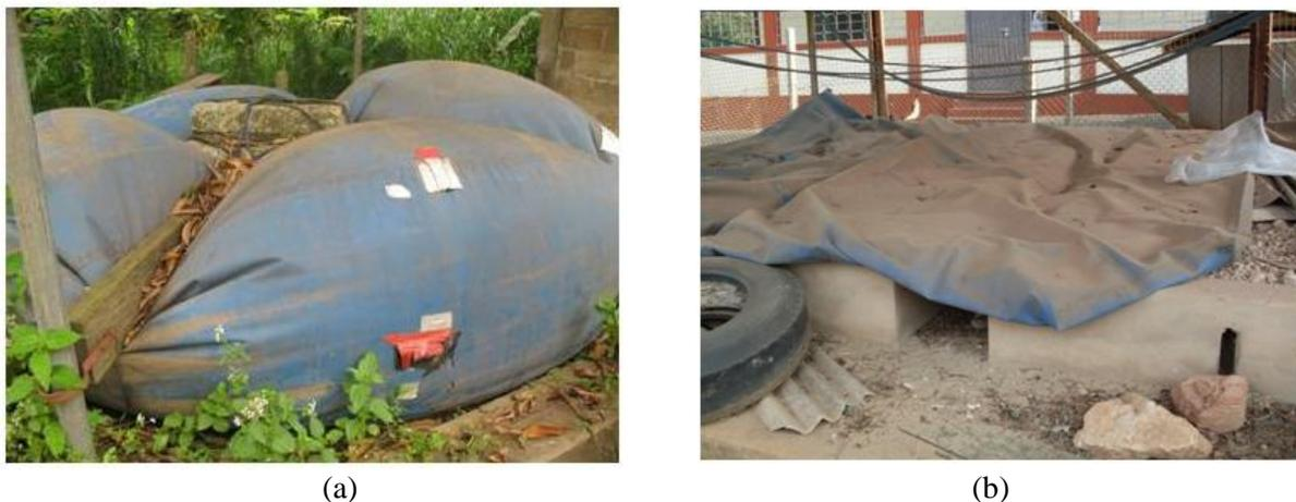
Figure 15. Deteriorated balloon gasholders at Holy Family hospital, Nkawkaw (a), June, 2008; and St. Dominic hospital, Akwatia (b), February, 2009
