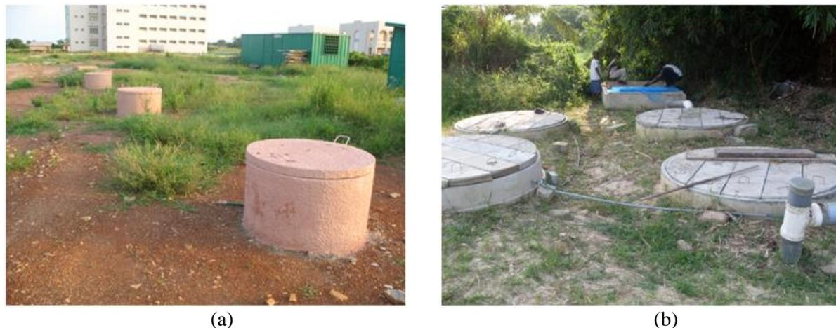
Figure 3. (a) Three 100 m<sup>3</sup> fixed-dome digesters at CUC, Miotso, November, 2008, and (b) Four 10 m<sup>3</sup> Puxin digesters at Hebron Prayer Camp, Hebron, November, 2008
